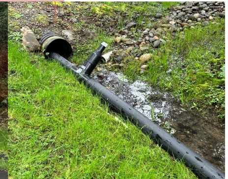
Sewer laterals temporarily rerouted as service lines are worked on
