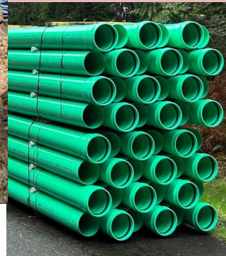
New service lines staged prior to installation
