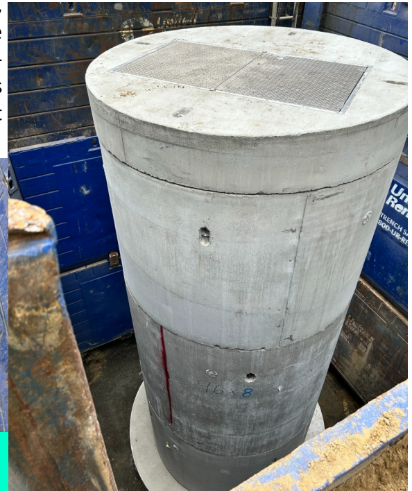
Above: Workers install the base for the new wet well Right: The wet well after installation
